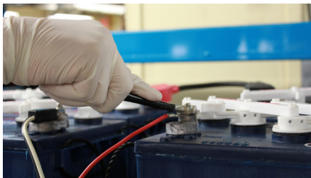
Figure 3: Remove positive lead from positive terminal on the battery pack
